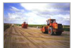
Road construction, F
