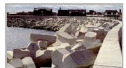
Marina construction, UK
